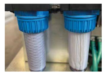
Double filter cartridge made of wound and pleated propylene, 10 microns and 1 micron respectively, to filter sediments from the incoming mains water. Sensors monitor the clogging status, indicating when replacement is required with a warning on the control panel.
